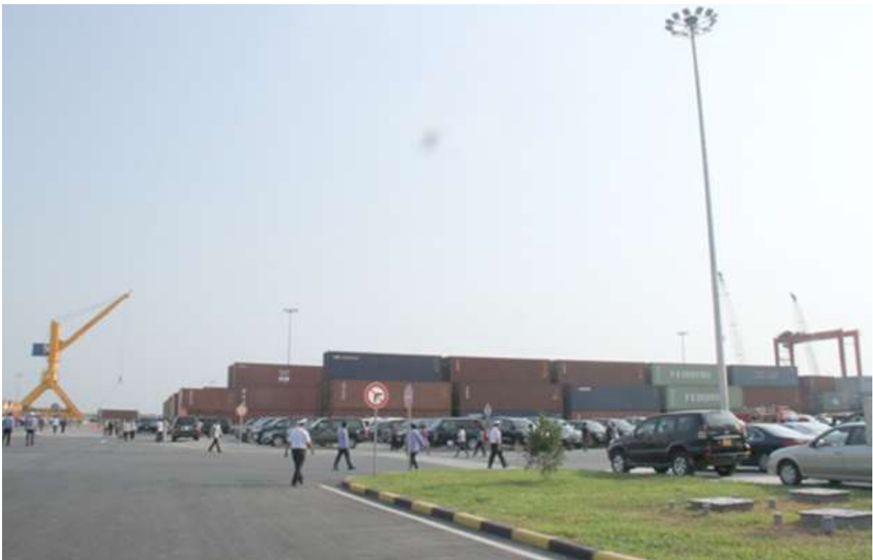
Kingdom's second largest new container terminal of Phnom Penh Autonomous Port in Kean Svay district, Kandal province. Photo: Chey Phoumipul
